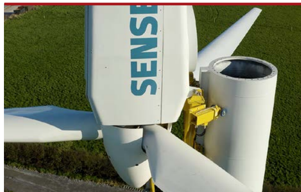
YOUR CARRIAGE AWAITS: The SenseWIND nacelle installation and removal technology in action on an onshore turbine
